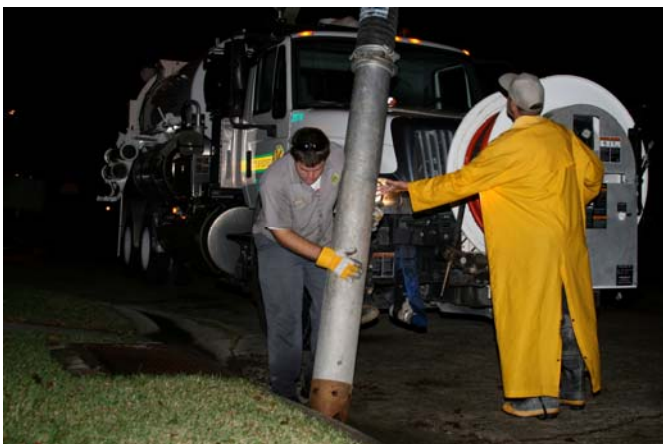
Kenner crew cleans street drain at 36 th & Arkansas Streets.]
